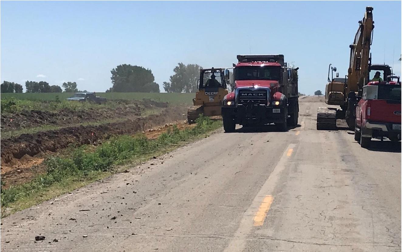
Shoulder work and smaller culvert work is being done by Fayette County Roads crews on the northern most end of W14 in preparation for a new asphalt overlay in 2021.
